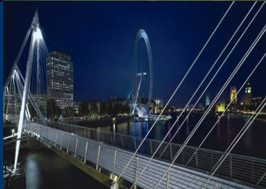
Golden Jubilee Bridge, London, 2002, WSP/Lifschutz Davidson, UK
