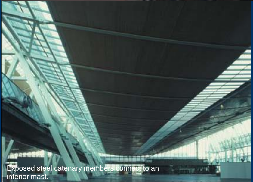
Dulles International Airport, Washington, DC, USA, Saarinen (Eero) and Associates, 1962. Inclined piers support the catenary slab.
